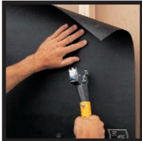
Staple 15 lb. roofing felt to 2" x 4" studs
