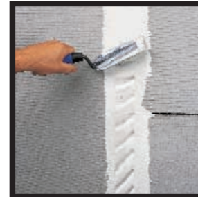
Tape panel joints
