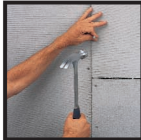
Simply nail using galvanized roofing nails
