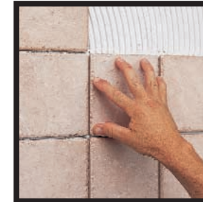
Press tiles into place
