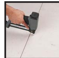
Fasten panels to wood floor
