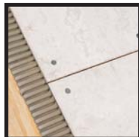
Adhere panels with mortar
