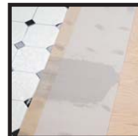
Vinyl flooring installation
