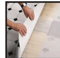
Install vinyl flooring
