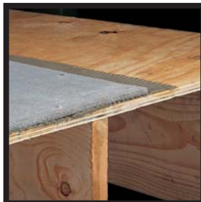
5/8" subfloor with 16" on center framing
